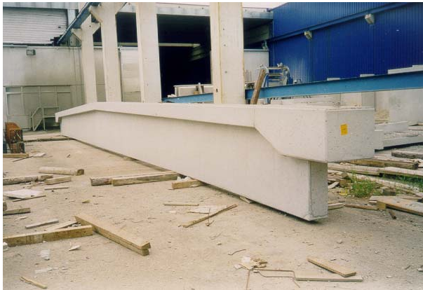
Fig. 1 Pre-fabricated reinforced concrete beam
