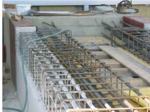
Figure 2: Reinforcement of a typically structural concrete beam
